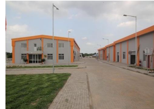
Solar Photo Voltaic Modules Manufacturing Plant in Mozambique
