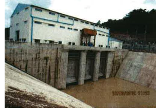
Small Hydro Project in Lao PDR
